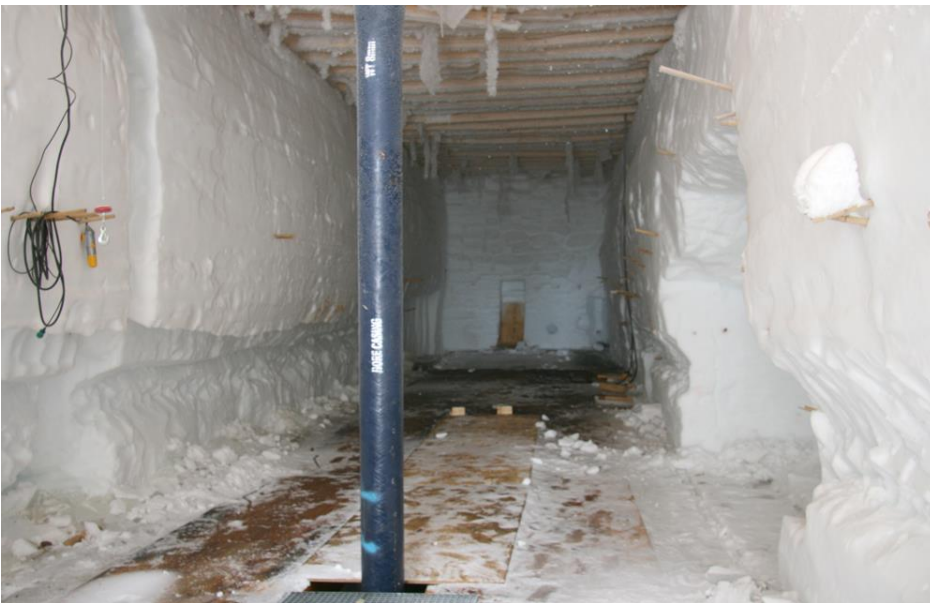
NEEM drill trench in 2012. Note the broken beams.
